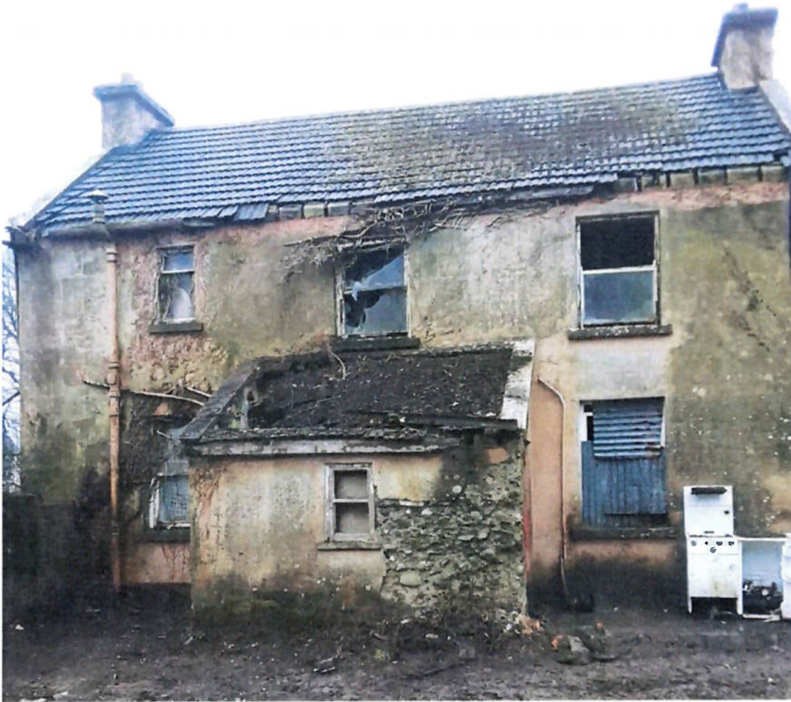
Recent Picture of rear of house before reroofing. Note concrete tile roof intact and soil vent pipe to first floor toilet.
